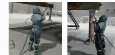
Actual application example at site
